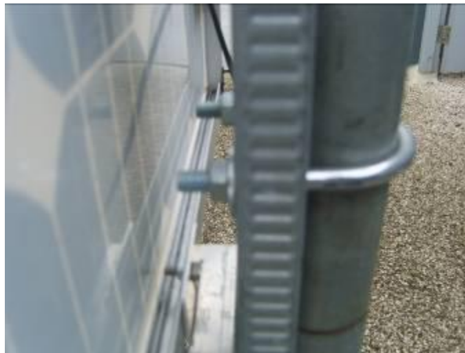
FIGURE 28 SOLAR PANEL MOUNTING HOLES BRACKETS
