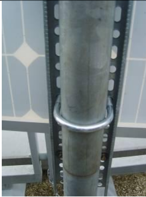
FIGURE 5 SOLAR PANEL MOUNTING HOLES AND U-BOLTS
